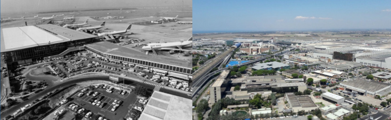
Aerial photo of the airport infrastructure, 1989 (left) and current (right)
